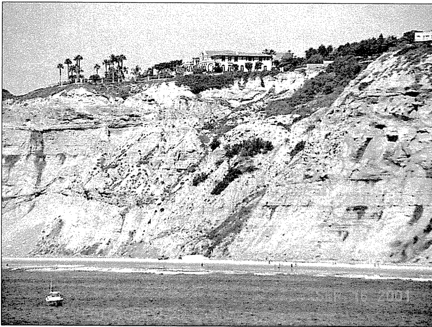
Seacliff failure north of Scripps Pier at Blacks Beach. Photo by Robert Hawk.
