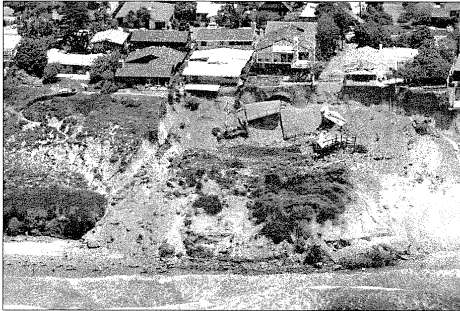
Coastal landslide, Leucadia, California, June 2, 1996. Photo by Michael W. Hart (Kendall L. Sherrod, pilot).
