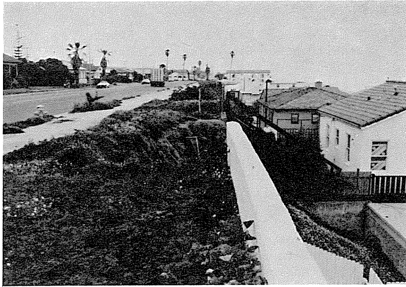
Figure 7 Ten feet of apparent slope retreat between two retaining wall structures. Eighteen inches of retreat are recorded after installation of gas pipeline.
