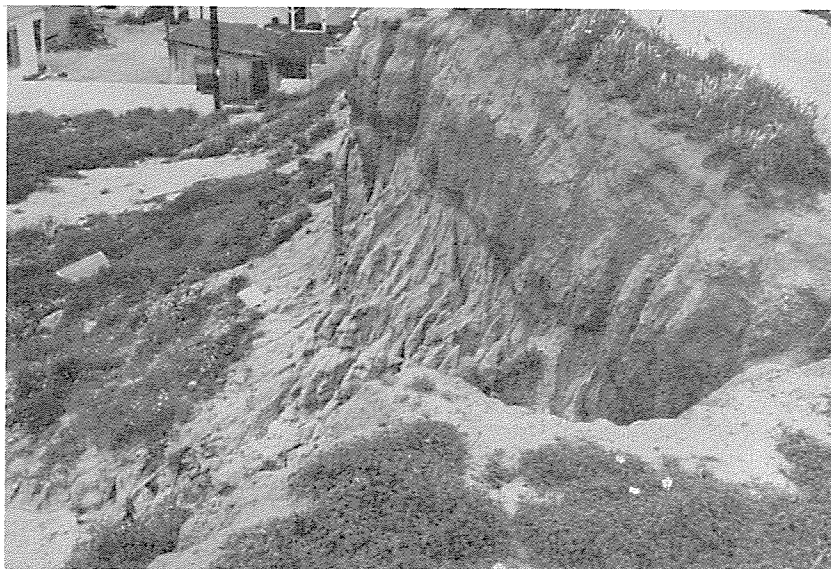
Figure 3 Geological conditions along a typical bluff segment viewed looking north from the proposed Tyson Street extension. Note the uniformity of the geologic units, slope inclinations and the general slope configuration.
