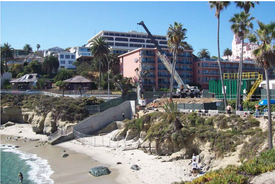
Caisson drilling for the new lifeguard station in La Jolla Cove
