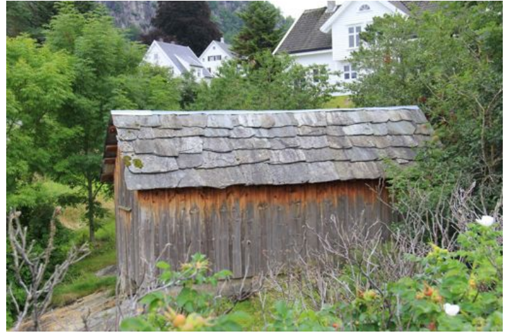
Slate roof on shed, Norway
